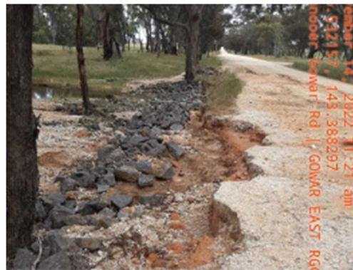
This road was damaged in 2011 (above photo) and again in 2018. It was damaged in the 2022 floods – shown in the right hand photo.
