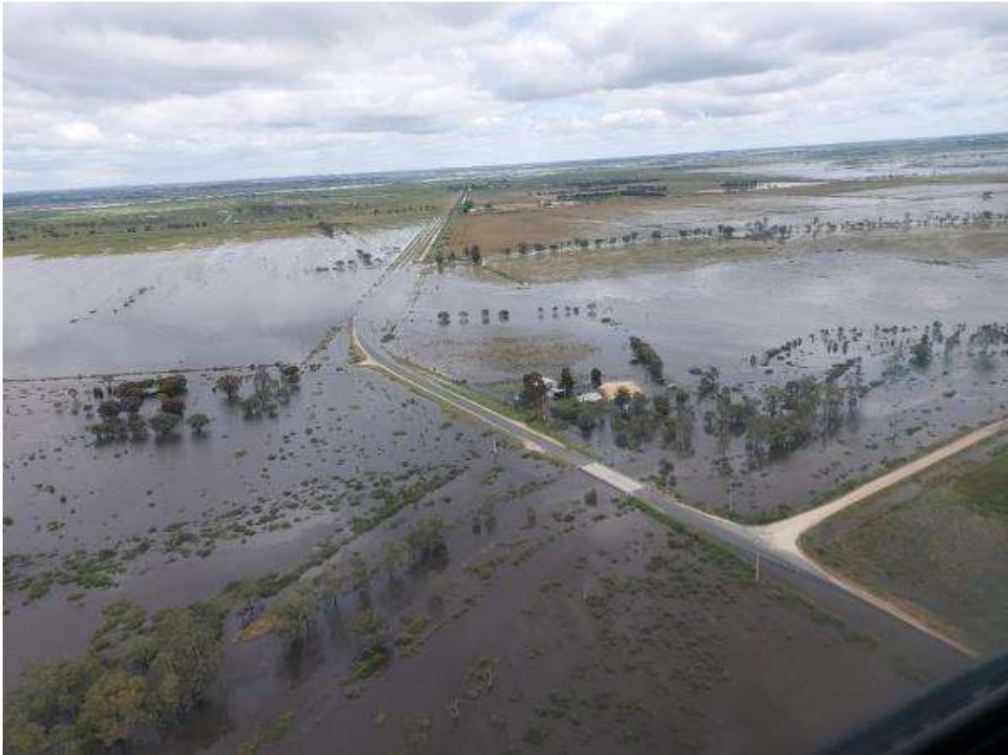
Unregulated flows from the Calival and Bullock Creek floodwaters crossing the Kerang-Koondrook Road at Sampson's Bridge
